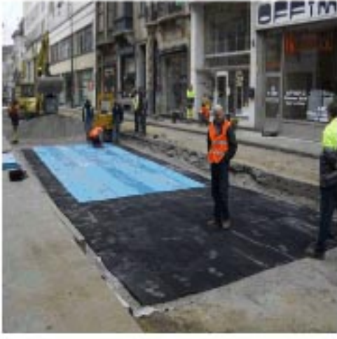
Installation of the resilient mat
