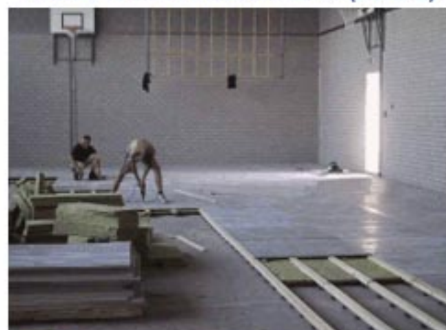
Installation of the floor
