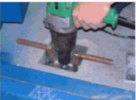
Jacking up the slab
