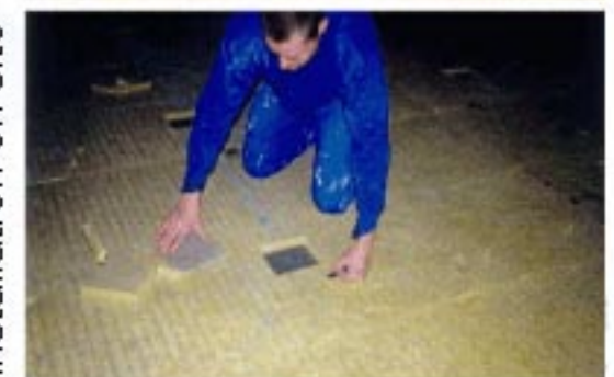
Installation on site
