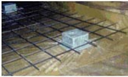
The boxes with reinforcement
